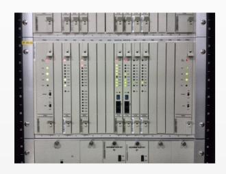
FA16 Multiplexer manufactured by H3C give us ground connections from Chengdu ACC to remote sites, for most remote sites, there are 2 different routes provided by different telecom provider.
